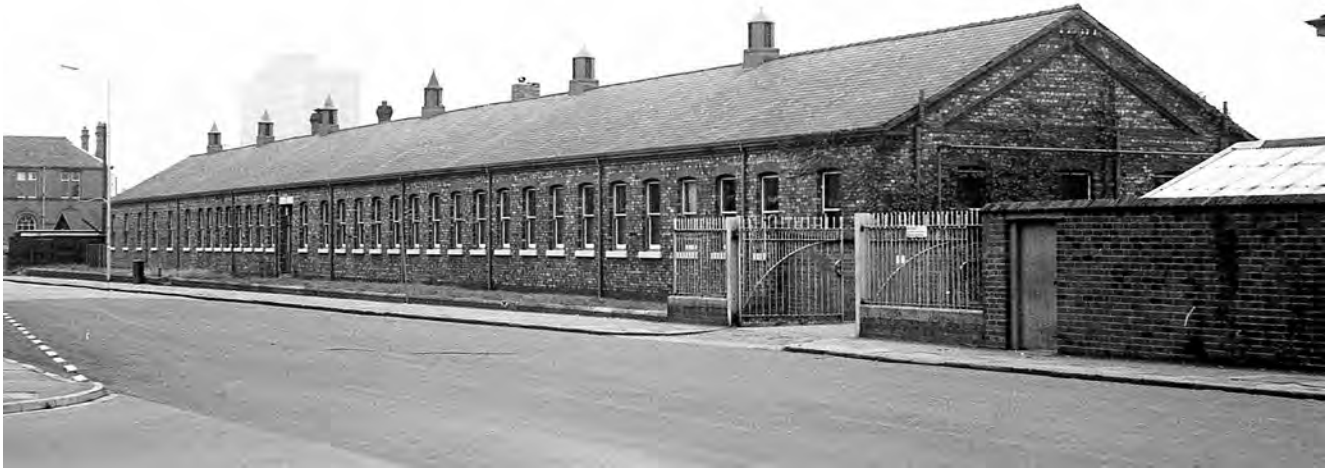
The LMS ex London & North Western Railway Signal and Telegraph Department offices at Crewe, built in 1903/4 and occupied by the then Signal and Electrical Department in 1904. The S&T workshops and stores were behind these offices.
