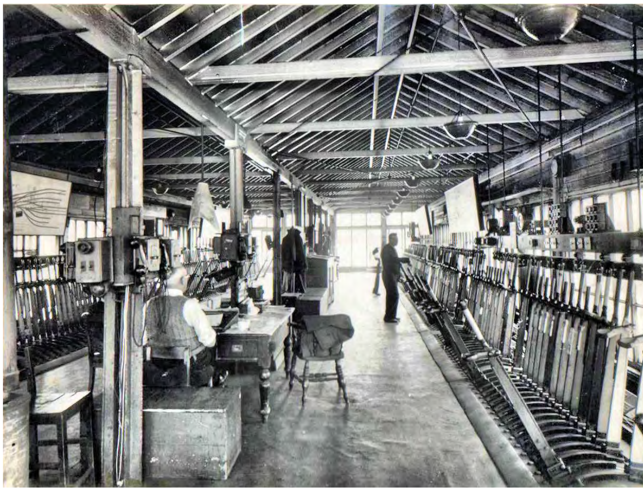
The interior of Euston No. 2 Signal Box.
