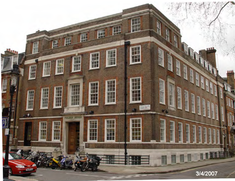
Plate 16. "Fielden House", 13 Little College Street, Westminster, built by the LMS for £48,961 in 1937.
