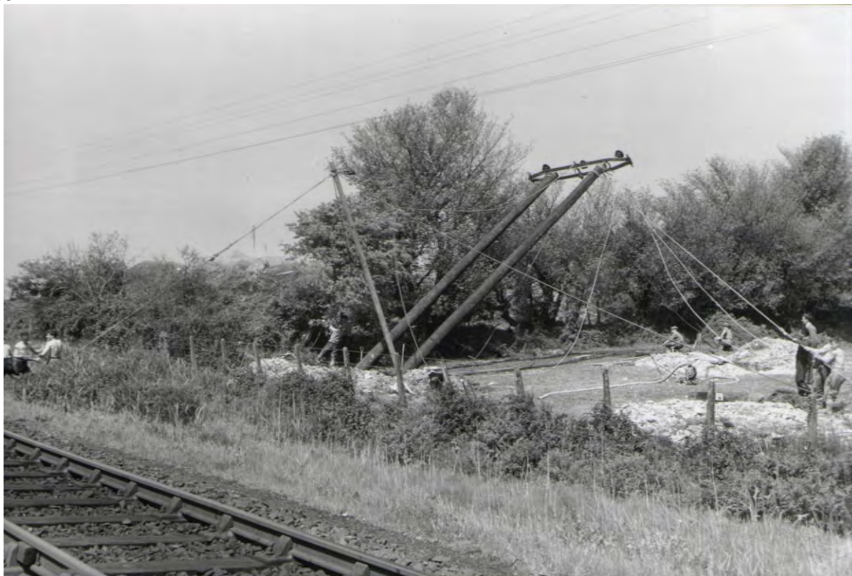
Somewhere on the Somerset levels an 11,000volt 'H' pole to Drawing SCGA 2/16 is being erected using a falling derrick. L. G. Warburton collection.
