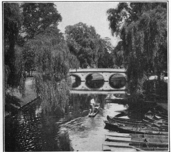
Trinity Bridge, Cambridge.
