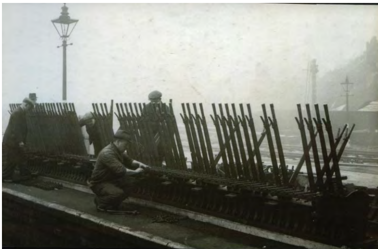
Erecting a new signal box Sheffield No.1.
