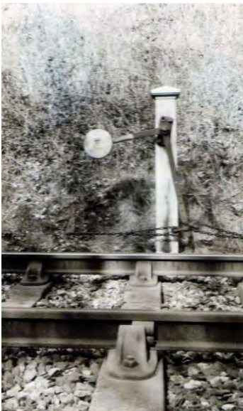
Plate 1. A gain stroke lever near Barnt Green on the line to Redditch and Ashchurch.
