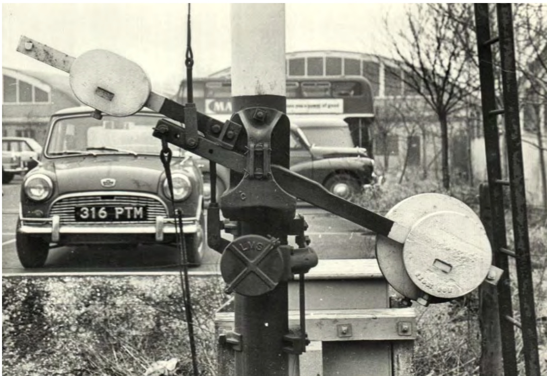
Plate 10. The LMS Standard slotting arrangement on a tubular post being Bedford St. John's Down Starting signal. This clearly shows the 'T' piece bolted to the upper distant arm balance lever on the left which stops the distant arm dropping 'off' by gravity until both levers in the signal boxes have been reversed..
