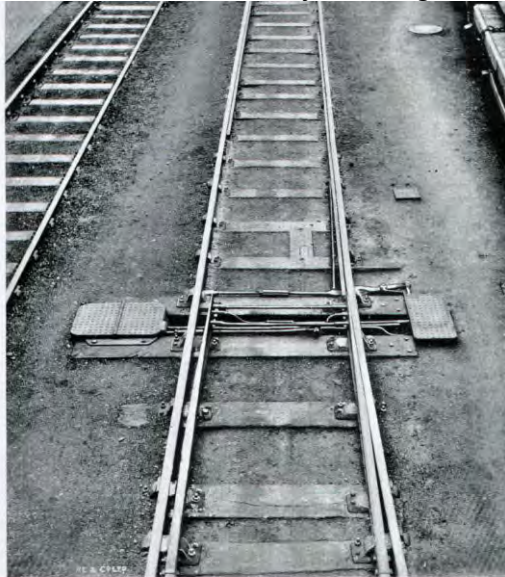
GRESTY LANE, CREWE, FACING POINT WITH MOTOR AND CHECK LOCK, &c.
