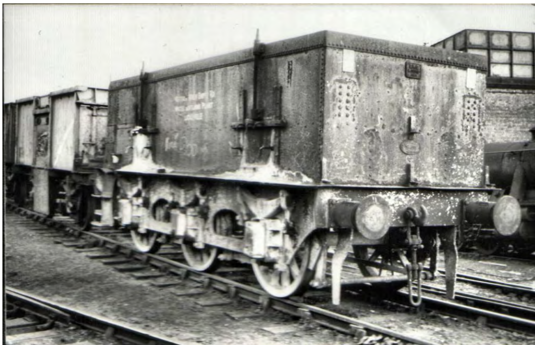
An ex Midland Railway Johnson tender, No.3047 built in 1924 and converted to a sludge tender at Coalville on 15 th September 1964.
