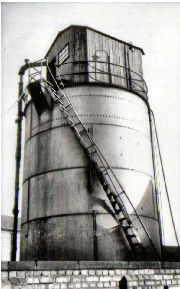
The far side of the Coalville softener showing the access ladder and the wooden building on the top of the tower.
