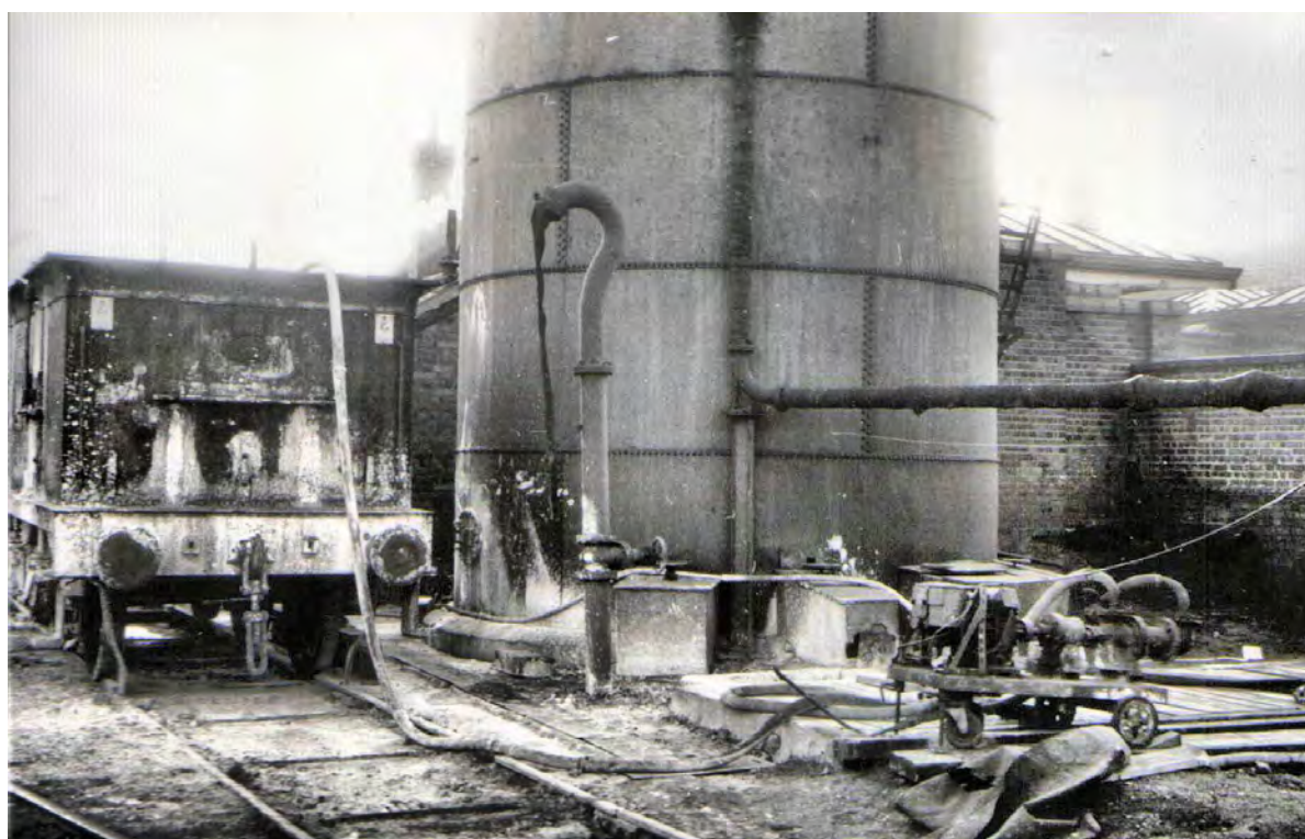
A close up of the base of the Coalville softener with a portable pump used to pump sludge into the adjacent ex MR tender.
